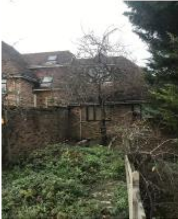
View of the existing dwelling from the south at Mid-terrace garden level
